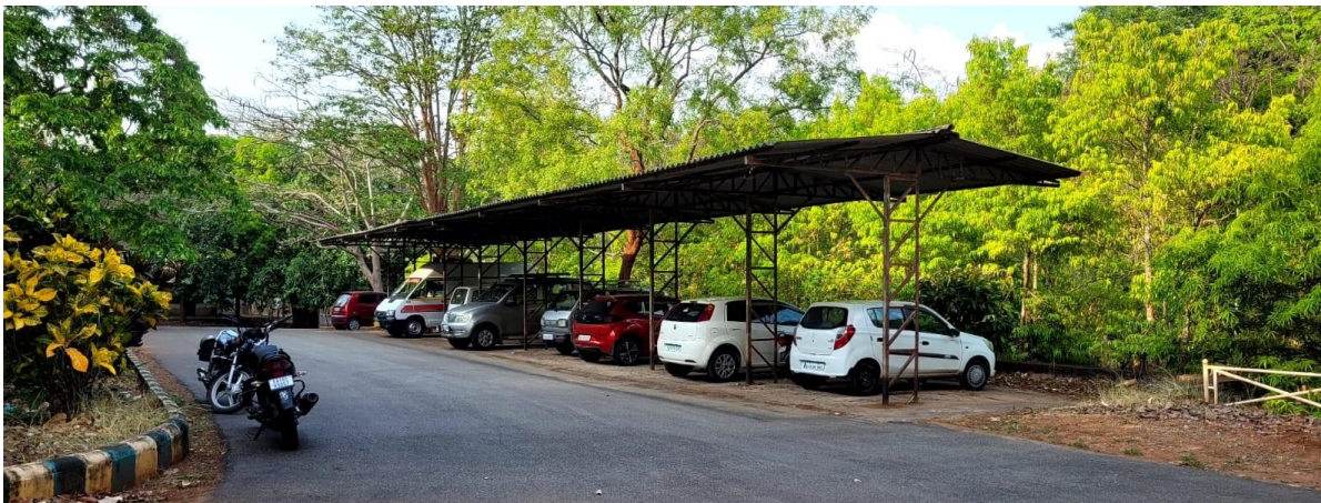
Fig 9.1: Parking shed near Arts Building
