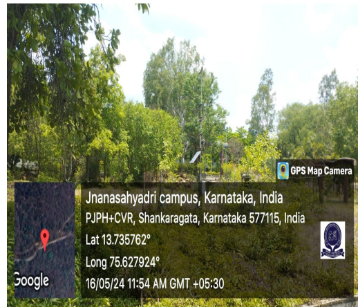
Wind energy unit at Pampavana
