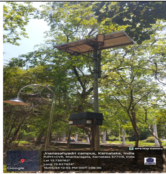
Solar Street light with LED bulb
