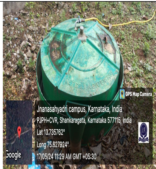
Bio energy production unit maintained in University campus
